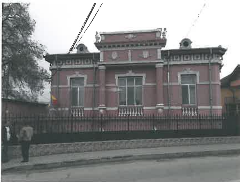
CONSTRUCTIA EXISTENTA C2
